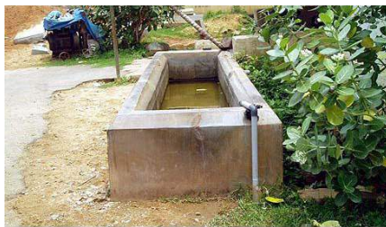
Fig 5.2: Low tank for cattle with drinking water pipe at entry
