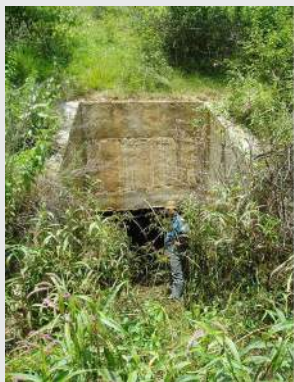
Fig g: Box-culvert: 5 to 6 feet high
