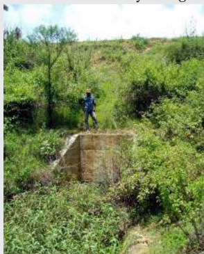
Fig h: Box-culvert lying 30 feet below overlying road
