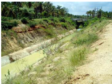
Fig 1.6: Channel after being lined with cement mortar
