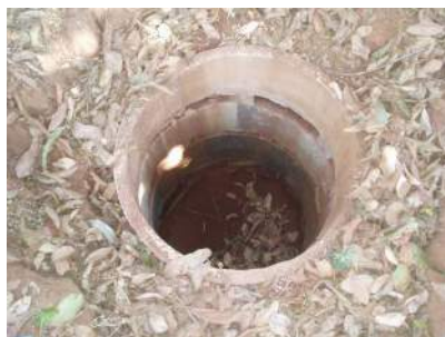
Fig 4.1: A six feet deep toilet pit encased with cement rings
