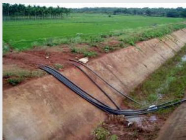
Fig. e: Low-lying area, channel lies above ground level with suction pipes placed in it
