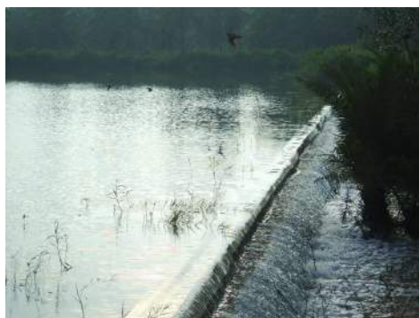
Fig 1.2: A tank's overflowing spillway
