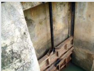
Fig. b: An escape gate with its attached screw visible
