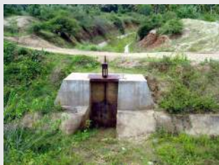
Fig a: An escape gate in a canal
